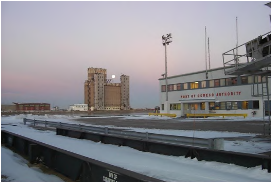
PHOTO 3 – 1998 looking West at West Pier Grain Elevator
